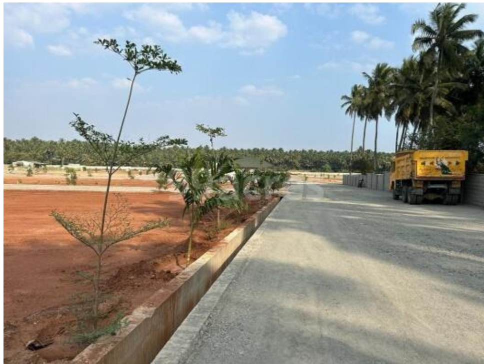
Development work in Kolkata Project
